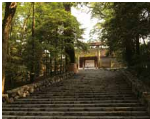
Main building of the Inner Shrine (courtesy of the author)
