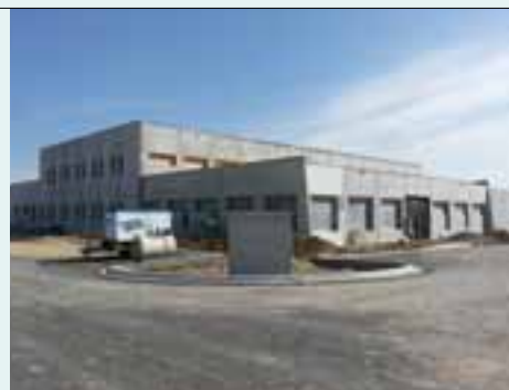
The new building under construction
