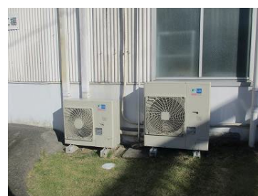
Cryogenic storage using alternative CFCs
