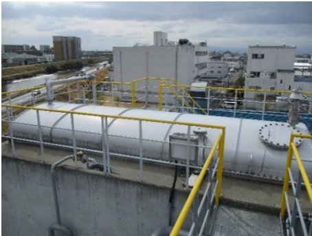
Wastewater treatment plant Anaerobic treatment tank
