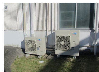
Cryogenic storage using alternative CFCs
